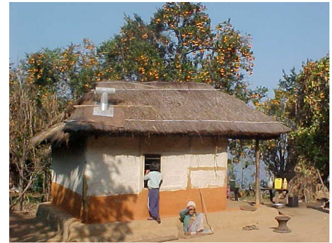
Chimney Pipe coming out of Kitchen roof
