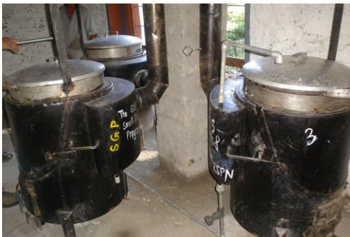
A set of newly installed fuel-efficient stoves in Nabji Community School
